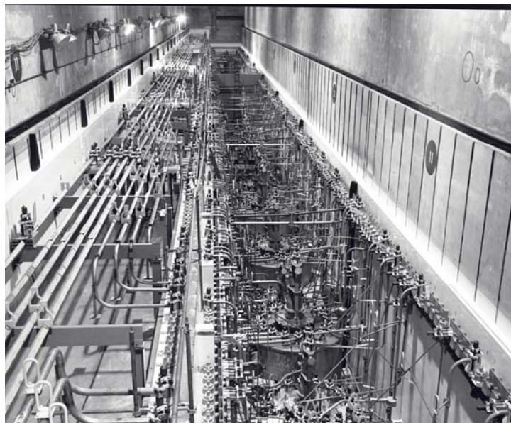
A “canyon” at Savannah River Site where the PUREX process was used to reprocess plutonium
